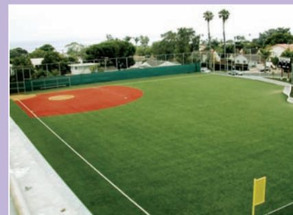
La Jolla High School has used artificial turf to provide a flexible-use field that can stand up to constant use.
